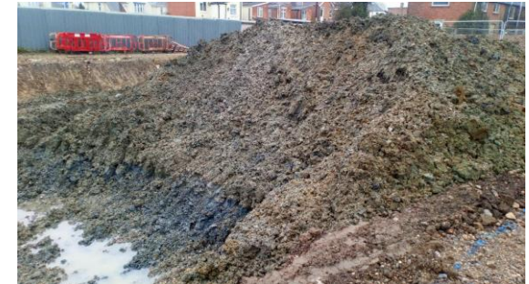
Figure 1: Excavation of hydrocarbon impacted material
