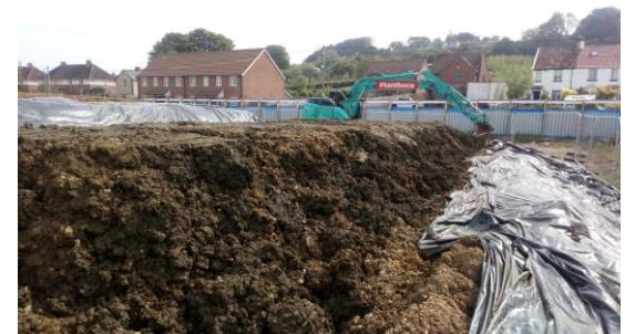
Figure 3: Windrows of impacted material within treatment area
