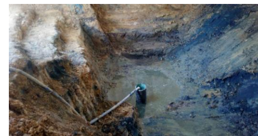
Figure 3 – controlled dewatering of the excavation.
