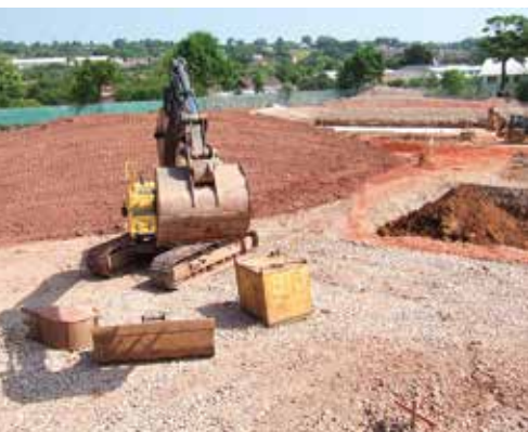
Delineated excavation of contaminated zones
