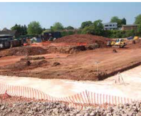
Re-profiling of site
