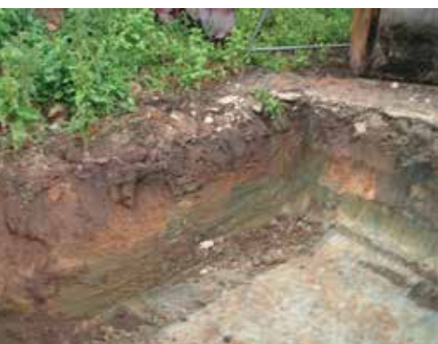
Completed tank removal excavation
