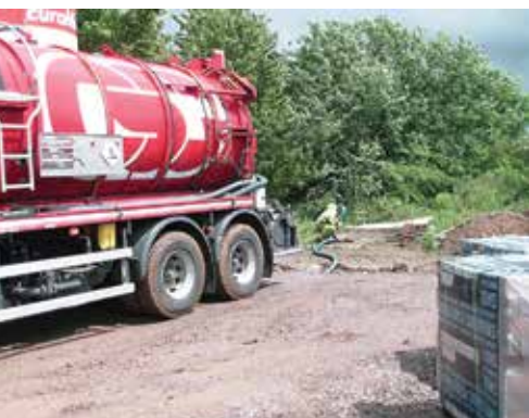
Tank being pumped out prior to excavation
