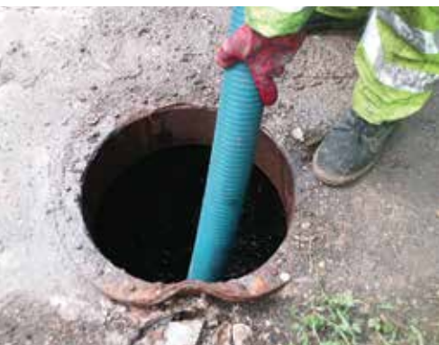
Tank being pumped out prior to excavation
