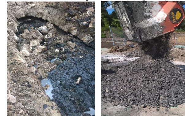
Hydrocarbon impacted organic sludge (left) was first dewatered in situ and then remediated using a stabilisation/solidification process.
