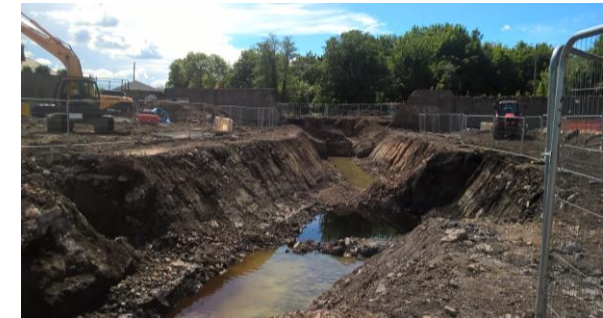
Hydrocarbon impacted organic sludge (left) was first dewatered in situ and then remediated using a stabilisation/solidification process.
